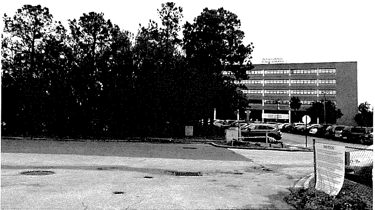
View of the subject site facing north with the School Board bldg on the right
